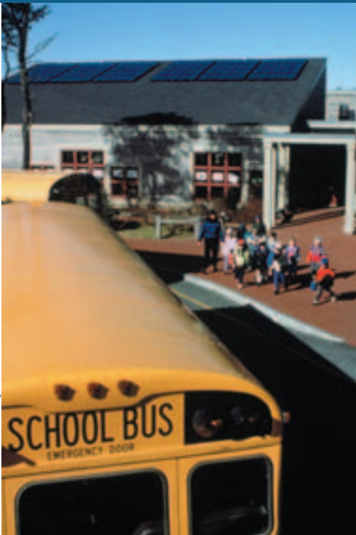
Nantucket Elementary School uses this grid-connected PV system.
