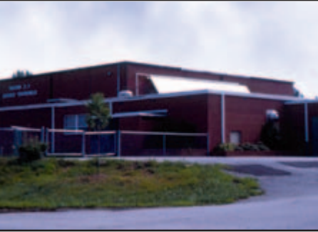
This solar domestic water system was added to the school's kitchen roof area and provides most of the hot water required by the cafeteria.
