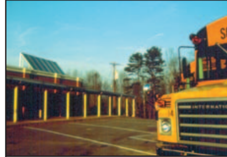
Photovoltaic systems in schools provide substantial energy savings and are educational tools for sustainability.
