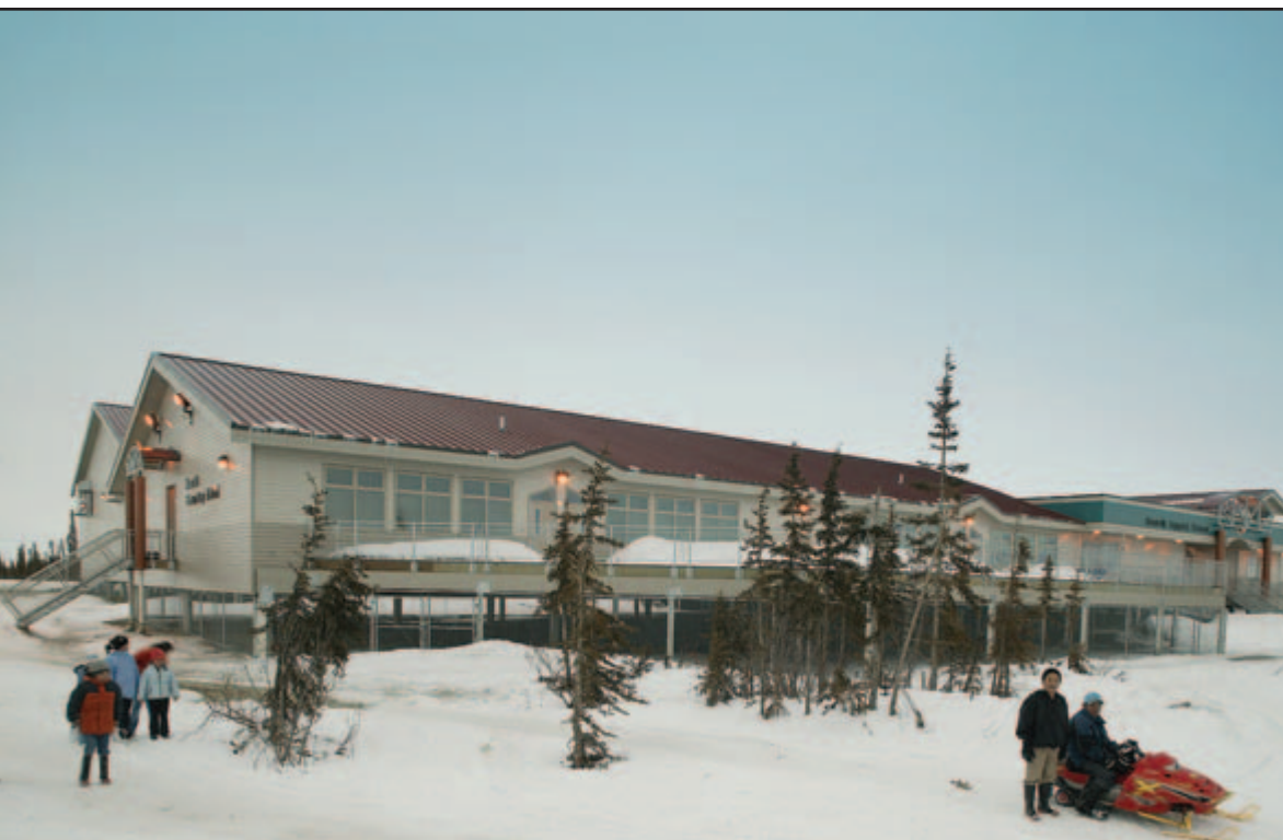
Photo: Krochina Architects
