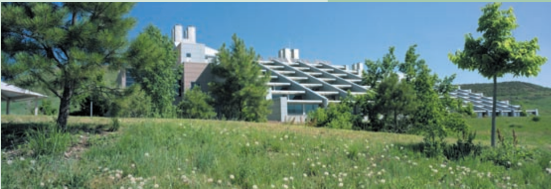
PIX 12618 Warren Gretz, NREL
