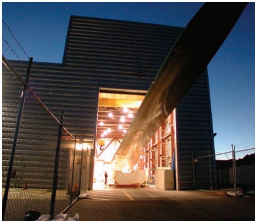
NREL is upgrading its blade test facility to provide industry with the means to test longer blades such as TPI's 45-m blade tested at the NWTC in 2004.
