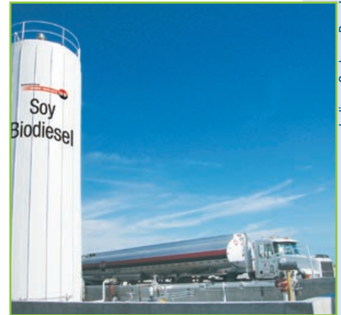
Pure biodiesel is stored in tanks like this and mixed with diesel to make blends of B2, B5, or B20.
