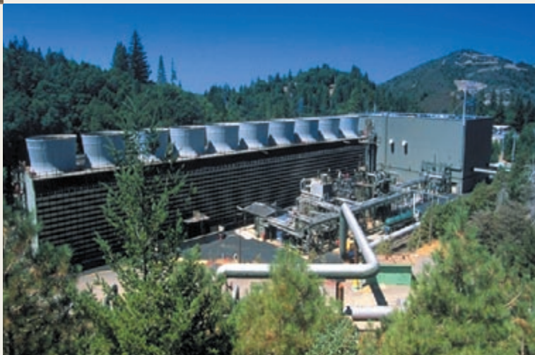
Pacific Gas and Electric Company (PG&E)
