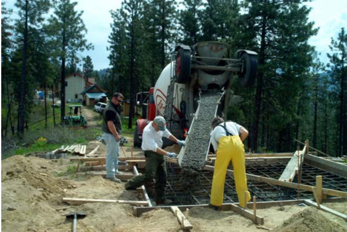
Figure 7: Foundation pad for Grim site. Source: NWSEED
