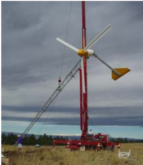
Figure 3: Bergey turbine being installed at Bassetti site. Source: NWSEED
