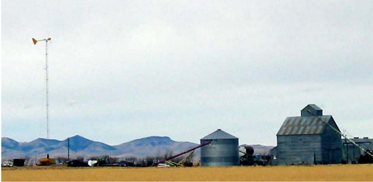
Figure 2: Turbine installed at Alger ranch in Stanford, MT.
