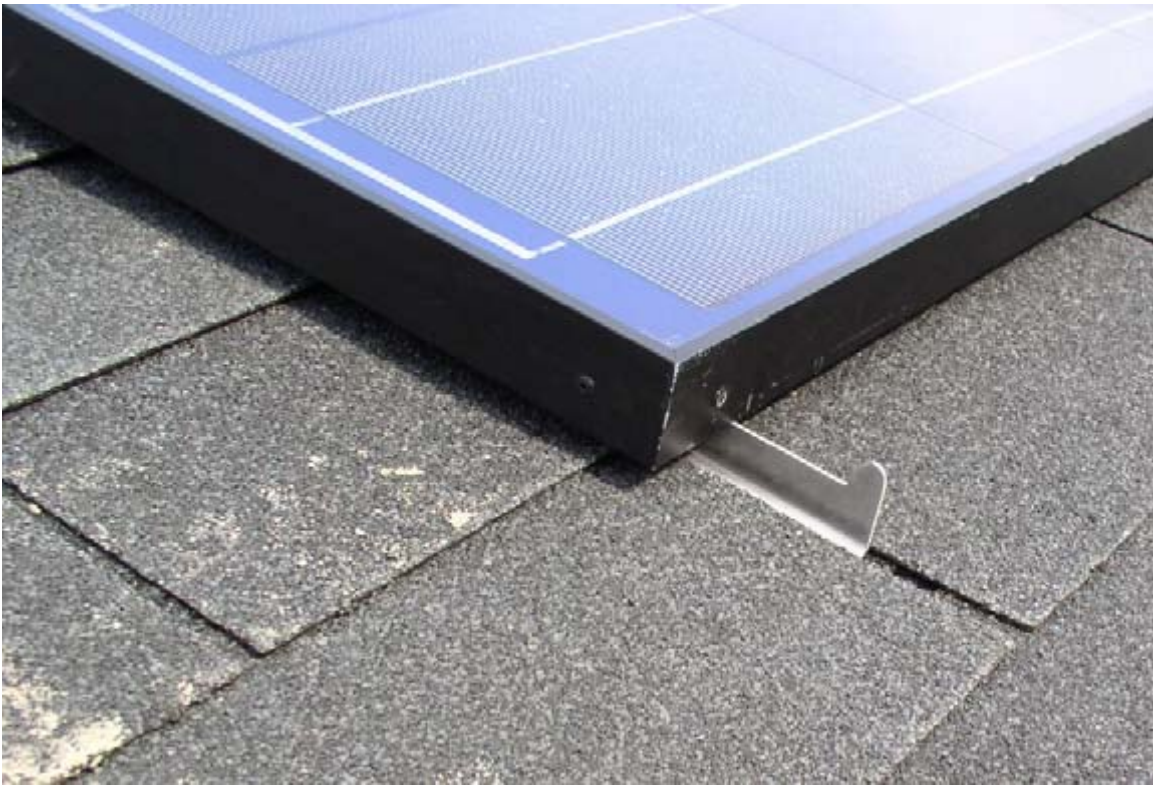
Figure 25. First APx-140 module installed on lower bracket.
