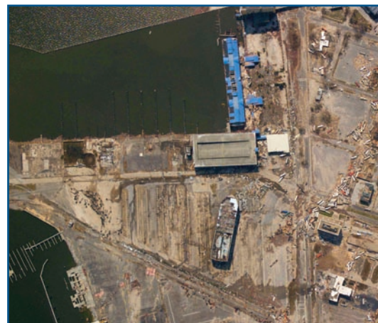
In 2005, Hurricane Katrina caused extensive damage to many industrial sites in the Gulf.
