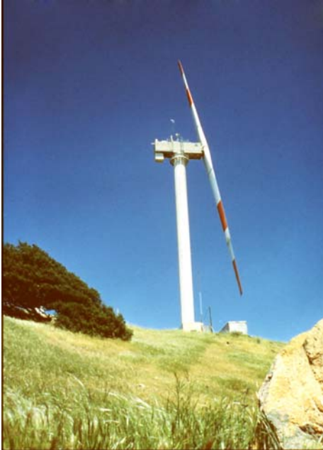
Figure1. The 3.2-MW Mod-5B, was the largest turbine in the Mod series.
