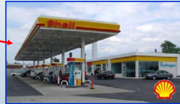
Hydrogen and gasoline station Washington, DC
