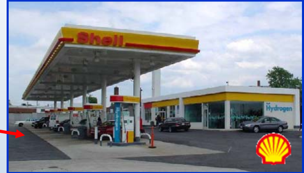
Hydrogen and Gasoline Station Washington, DC
