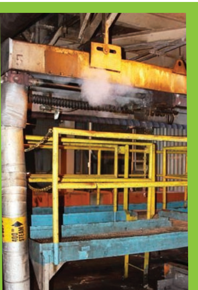
After the assessment, the mill was able to reduce the steam used by its soot blowers, like the one pictured here, by 40%.
