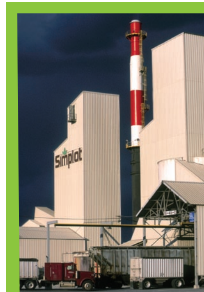
The J.R. Simplot Company's Don plant, located in Pocatello, Idaho, produces more than 1 million tons of phosphate fertilizers, feed phosphates, and related industrial products annually.
