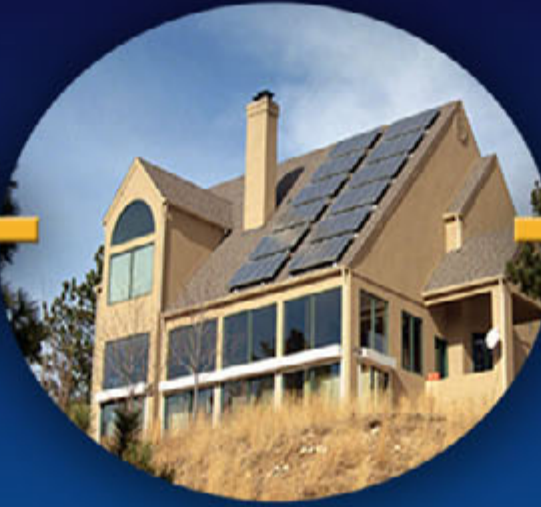
Energy Smart Buildings
