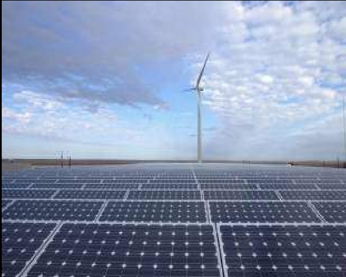
WorldWater & Power and Alternity Power Atlantic County Wastewater Treatment Plant, 8 MW solar-wind hybrid, NJ
