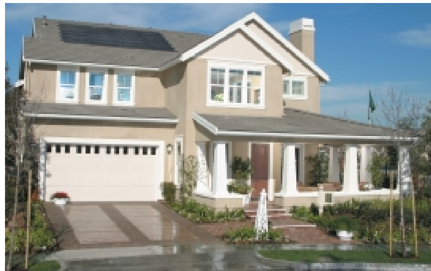
Notice the latest generation of solar panels on one of the Terramor homes. (Photo courtesy of Shea Homes.)
