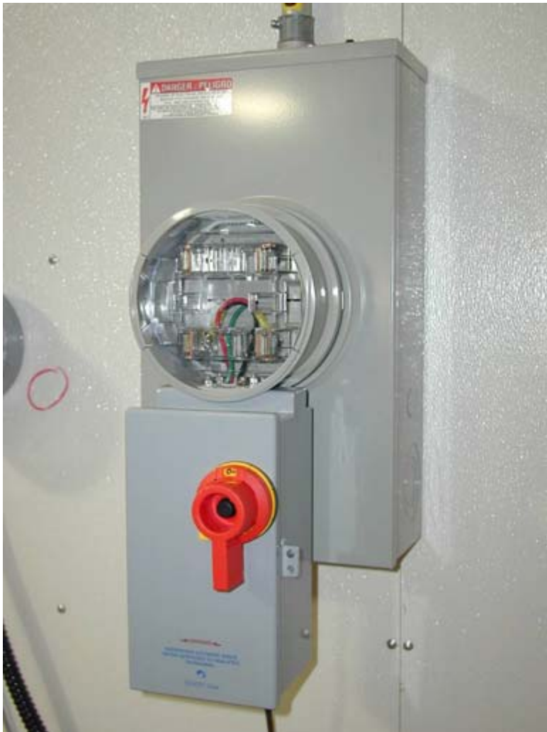
Fig. 2-8a and 2-8b. To use the Meter Interconnect Device with a ringless style meter socket, there is a second, shallow extender that goes in place first. The bottom photo shows the MID in place with a ringless meter socket.
