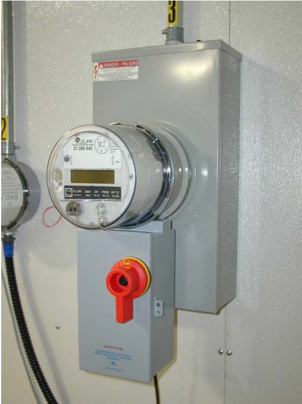
Fig. 2-9. The Meter Interconnect Device installed in a ringless style meter socket.
