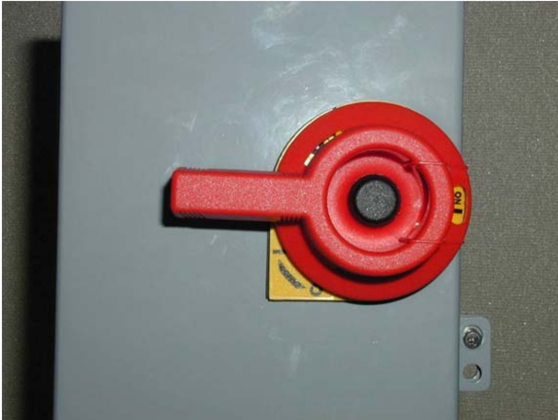
Fig. 2-4. The switch handle is shown in the “on” position, which prevents the door from opening. Rotating the switch handle 90 degrees ccw into the “off” position allows the switch to be locked and the door to be opened. A captive fastener secures the hinged lid. A spare hole in the tabs is provided for a padlock or tag.
