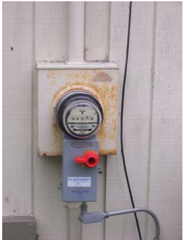
Figures 2-13 and 2-14. The residential PV system installation in Lanesboro, MA.
