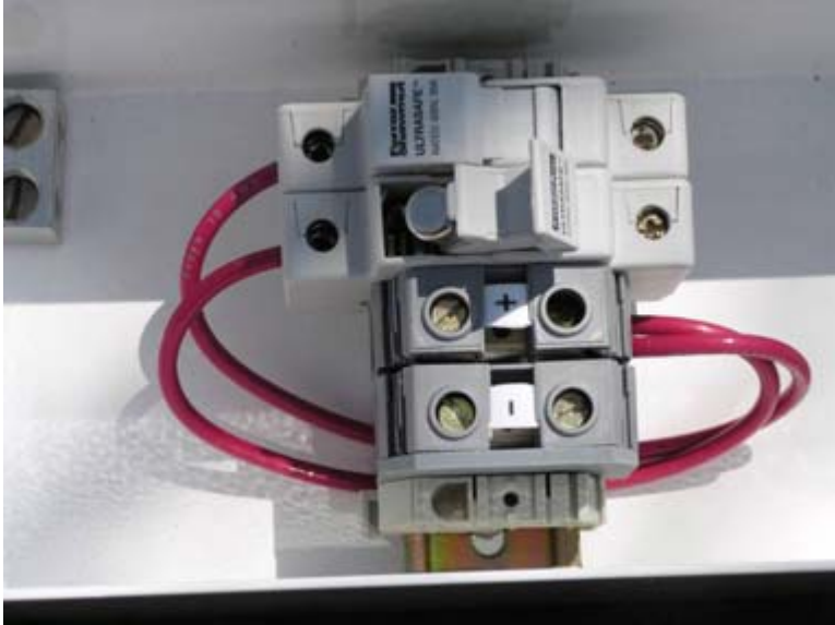
Fig. 7-7. Terminal blocks for the PVSCP 2F/150. Terminals are mounted on a rail secured to the bottom of the enclosure. Fused blocks accommodate up to 30amp fuses. When popped open (as shown in lower fuse block) the fuse is isolated from live circuits and safe to remove.
