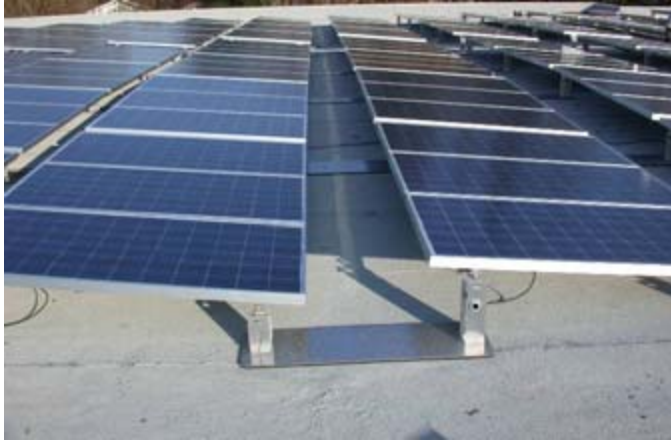
Figure 4-7. View of baseplate with both RoofJacks supporting PV module assemblies.
