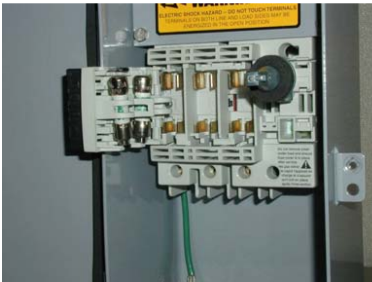
Fig. 2-3. The black C-shaped handle (see Fig. 2-2) opens the fuse door in the switch, allowing safe access to the fuses for convenient and safe insertion, inspection or replacement.
