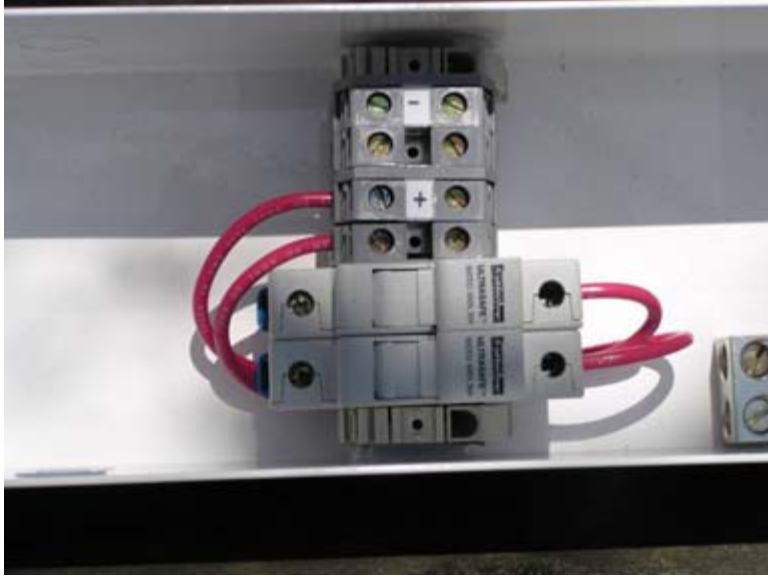
Fig. 7-8a,b. Terminal blocks for the PVSCP 2F/65 (top photo) and PVSCP N/150 (lower photo) are shown.
