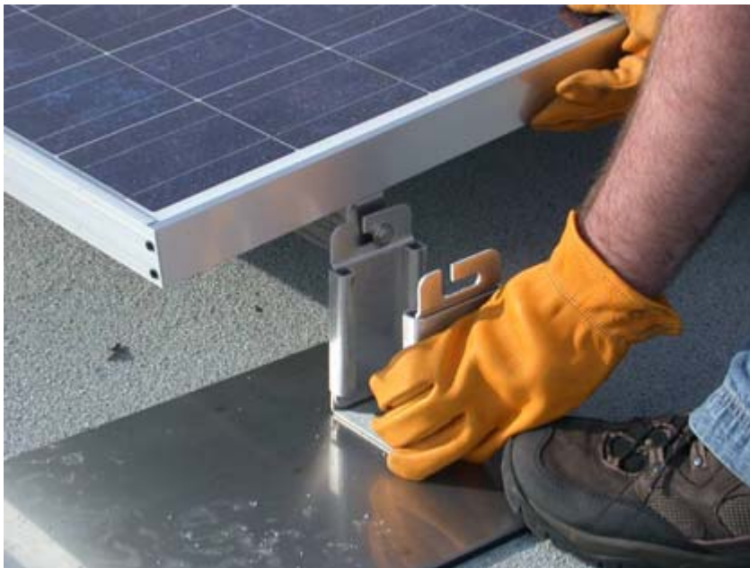
Fig.4-8. Panel assembly resting in the lower RoofJack
