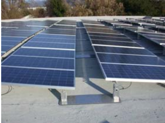
Figure 1. The free-standing (FS) system developed under this contract is the flagship PV array mounting system offered by the company. Wind-tunnel testing and extensive analyses were made possible by the project to help establish the applicability of the FS mounting system.
