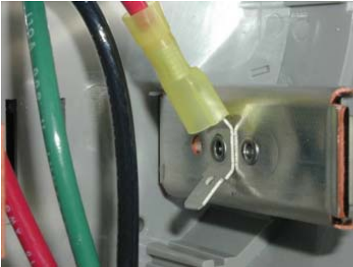
Fig. 2-6a and 2-6b. Factory wiring emanates from the output of the fused switch and passes through a hole in the enclosure and meter extender. The meter extender is equipped with spade terminals riveted in the factory to the metallic sockets. The ac wiring from the switch is factory wired to these spade terminals in the meter extender.
