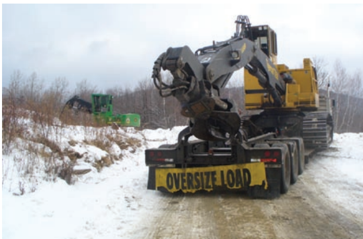
Road construction begins on the Lempster Wind Project. (Photo credit: Iberdrola Renewable Energies USA/PIX15574)
