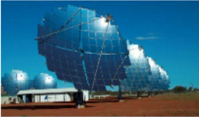
Dish: requires active cooling
