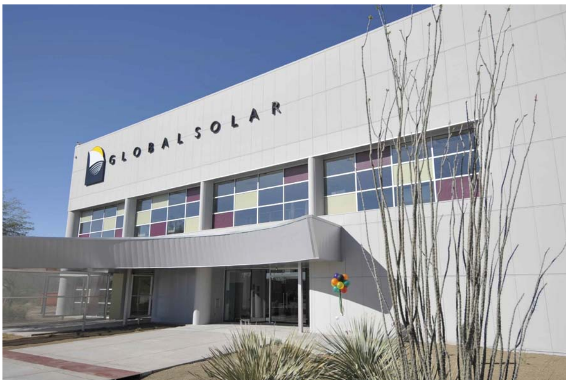
Figure 2.1. The new Global Solar Energy manufacturing facility in Tucson (10,220m 2 ).
