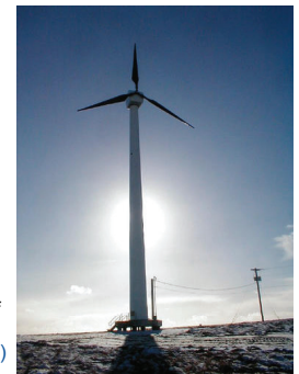
Three Northern Power Systems Northwind 100/19 (100-kW) on special permafrost foundations.
