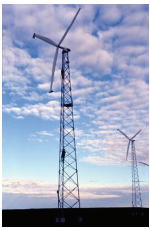
Kotzebue, Alaska Wind Farm consisting of 15 AOC 15/50 or Entegriy EW50 (50 kW); one Vestas V17 (65 kW); and one Northern Power Systems Northwind 100/19 (100-kW).
