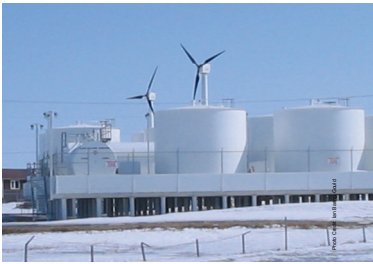
NW100 turbines over bulk fuel tanks in Kasigluk, Alaska.
