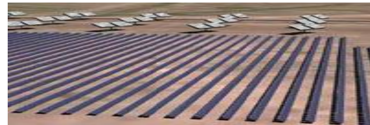
8MW PV Plant, Alamosa, CO
