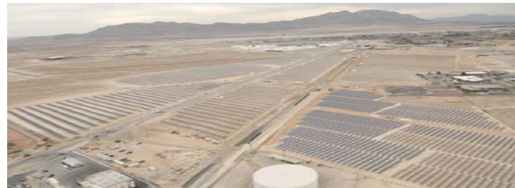
14MW PV Plant at Nellis AFB, NV (largest PV plant in the North America)
