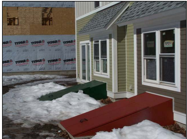
Figure 4. Hatch door to basement stairway
