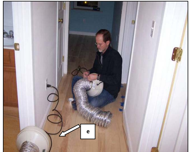
Figure 18. Mixing fan and duct setup
