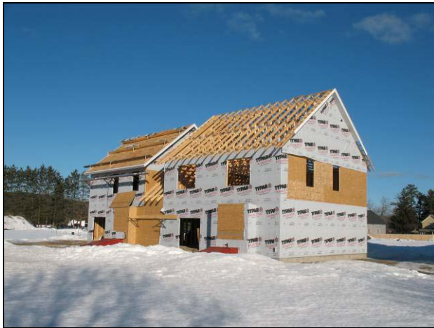
Figure 3. Adjacent duplex under construction
