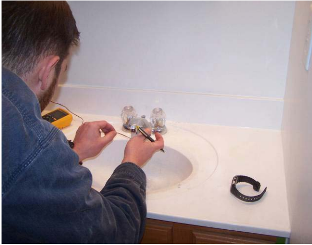
Figure 39. Hot water draw test
