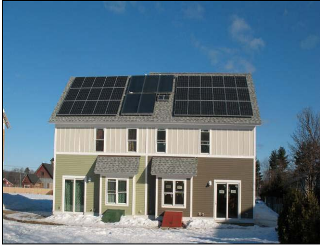
Figure 1. Back south view of the duplex building
