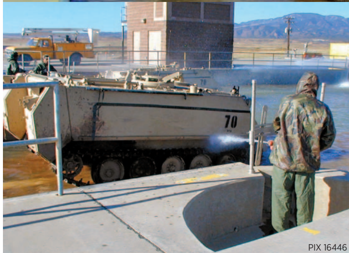
Soldiers hose down trucks with high-pressure water to clean off debris in the Fort Carson Central Vehicle Wash Facility. The basin, known as a “birdbath,” collects the water for reuse.
