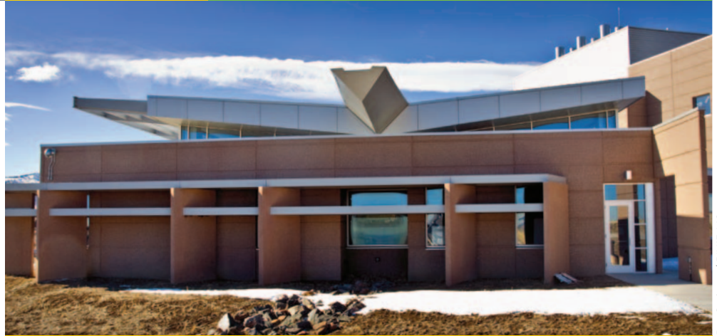
The Science & Technology Facility at the National Renewable Energy Laboratory in Golden, Colorado, incorporates a number of advanced energy efficiency and green building concepts. For example, the architecture makes good use of natural light wherever possible, and an automated system dims unnecessary artificial lighting to reduce electricity use.
