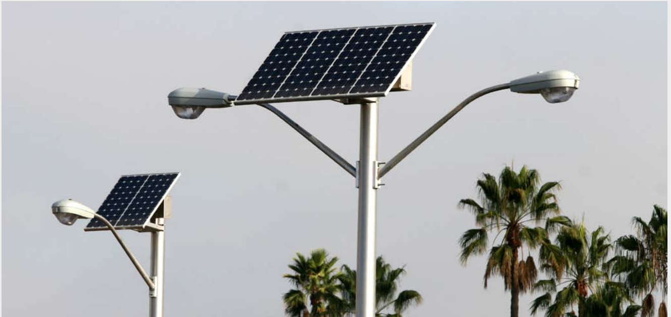
One energy conservation measure implemented by MCAS Miramar is solar-powered parking lights. The Secretary of the Navy awarded MCAS Miramar the 2009 Energy and Water Management Award.
