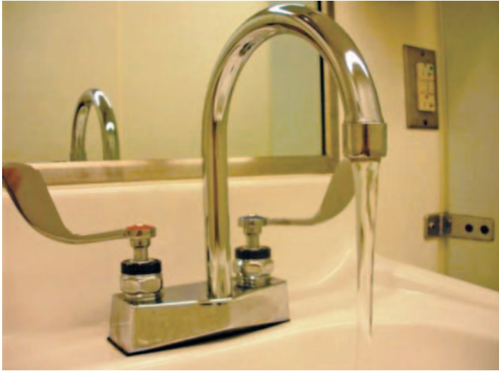
Laminar flow faucet in Huntington VA Medical Center
