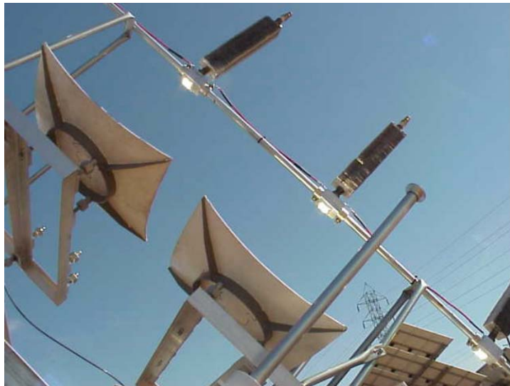
Fig. 3.1.4 Concentrator cell assemblies in the Arizona Public Service (APS) STAR facility.
