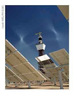
Concentrating solar power (CSP) technologies, such as power towers, are potential demonstration projects for the Solar Demonstration Zone in Nevada.
