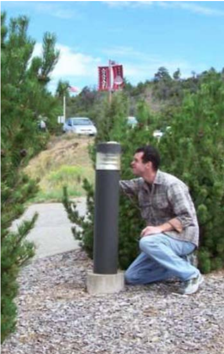
BLM replaced exterior lighting with energy-efficient models.
