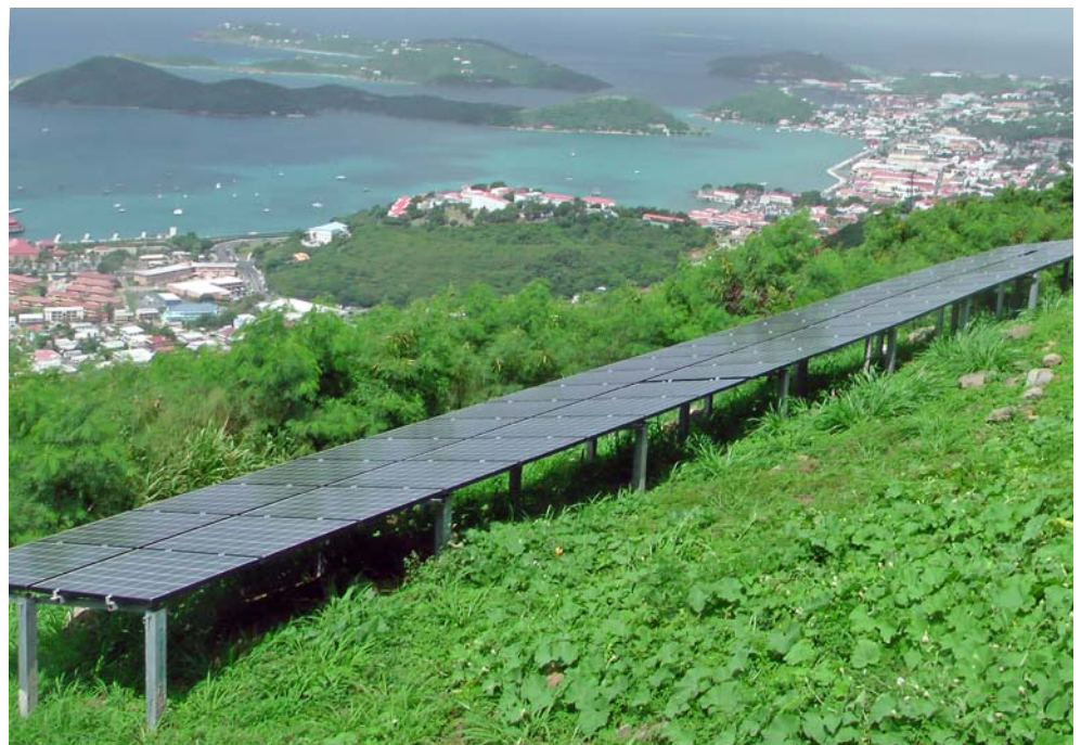
Many Virgin Islands residents have taken advantage of rebates offered through VIEO for renewable energy systems. This 10-kW PV system is located on Skyline Road on St. Thomas, overlooking Charlotte Amalie. Photo from Don Buchanan, VI Energy Office
