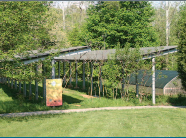
The Solar America Cities program provided funding to enhance a solar energy exhibit at the Ijams Nature Center, near downtown Knoxville. Photo from City of Knoxville, NREL/PIX18694
