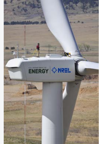
The DOE-GE 1.5-MW wind turbine is 80 meters tall and has a 77-meter rotor diameter. Photo by Dennis Schroeder, NREL/PIX 19083
