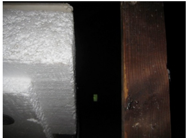
Figure 13. Left: Corner of attic access hatch insulation dam and frame; Right: Attic hatch insulated but without gaskets
