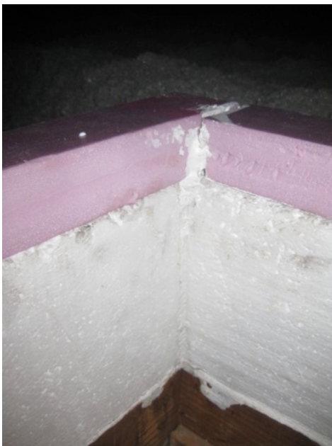
Figure 13. Left: Corner of attic access hatch insulation dam and frame; Right: Attic hatch insulated but without gaskets
