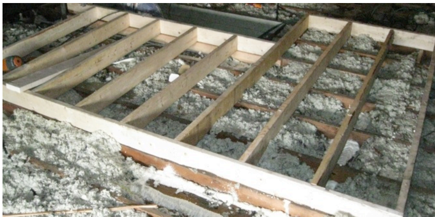
Figure 15. Storage platform framing (Photo credit: S. Marchese, printed with permission)
