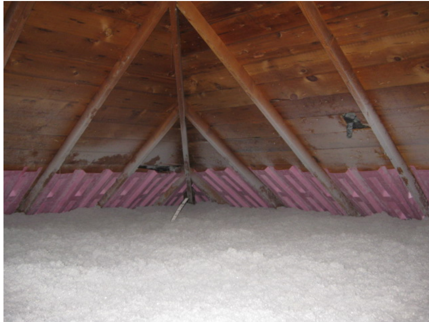
Figure 17. Vent chutes used to block cellulose from filling roof soffit
