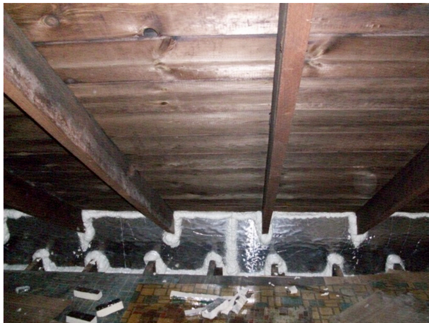
Figure 5. Foil-faced polyisocyanurate insulation board with seams and joints sealed to adjacent framing
