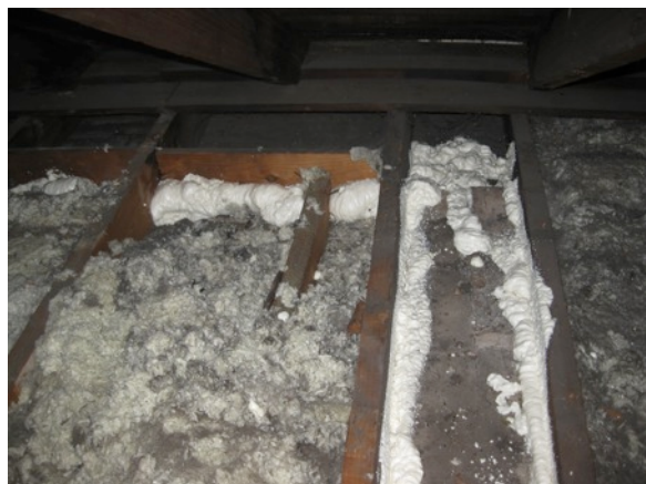
Figure 9. Left: Creating access to dropped soffit area and plumbing wall; Right: Attic floorboard repurposed in sealing plumbing chase (Photo credit: S. Marchese, printed with permission)
