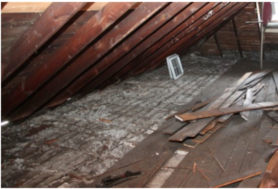
Figure 8. Left: Attic floorboards partially removed for attic deck air sealing and insulation; Right: Attic floorboards removed intact (Photo credit: S. Marchese, printed with permission)
