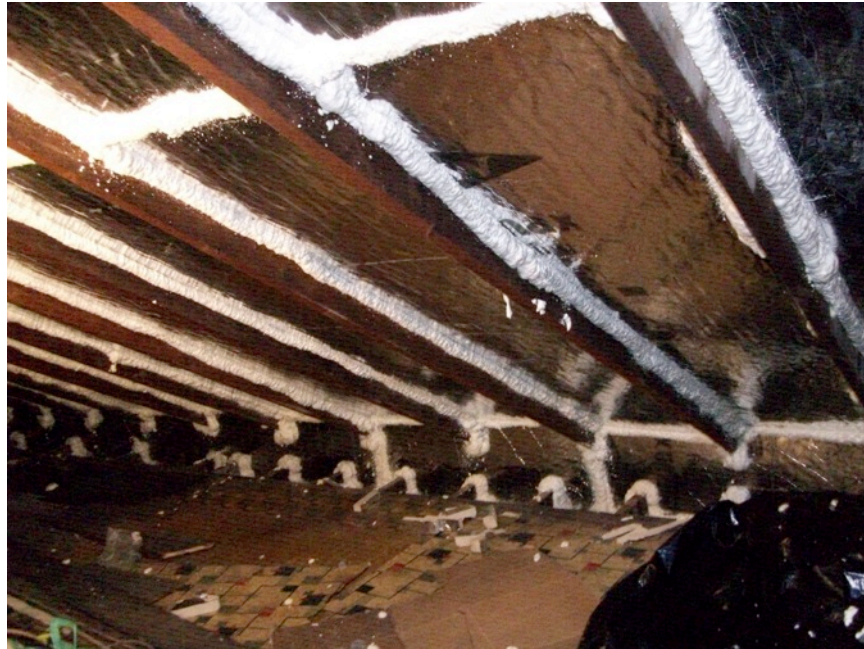
Figure 6. Foil-faced polyisocyanurate insulation board between roof rafters and transitioning to top of wall with seams and joints to adjacent framing sealed
