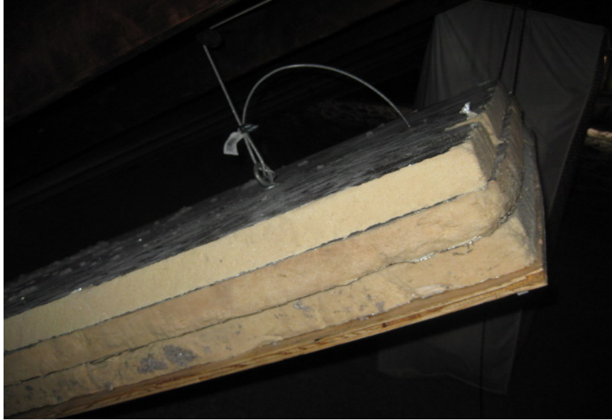
Figure 14. Hinged attic hatch with counterweight over attic access stairs. Gaskets and weather stripping are located on the stationary frame.
