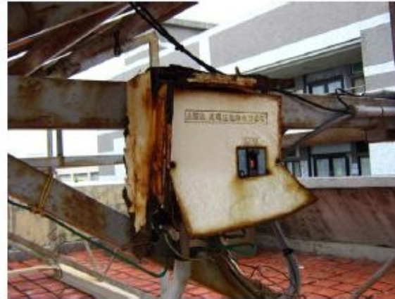
Corrosion in a harsh environment
