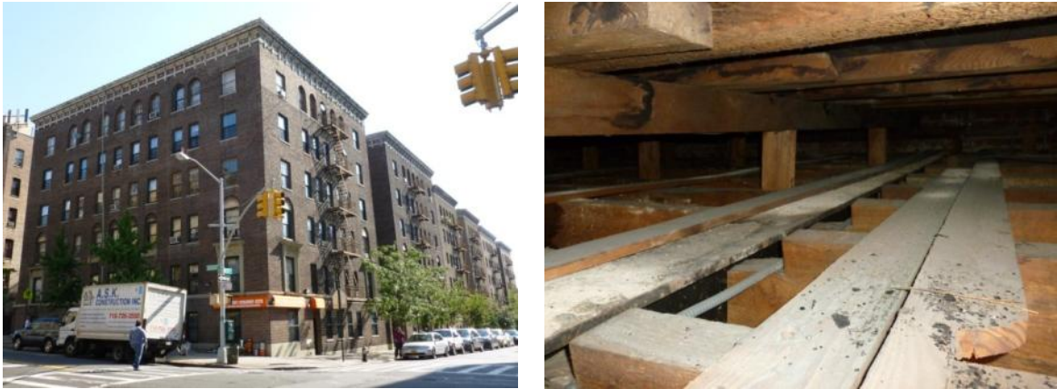
Figure 45. Attic space typical of this type of building
