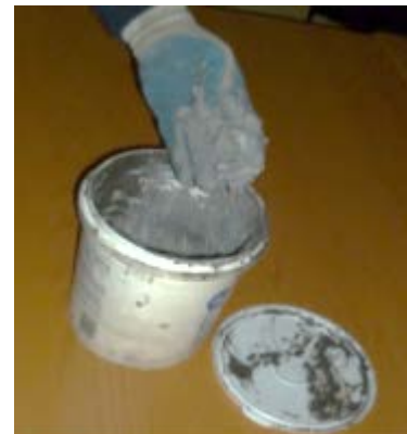
Figure 21. Mastic can be applied with a gloved hand
