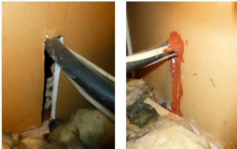
Figure 40. Process of sealing a hole in a fire-rated assembly between apartments
