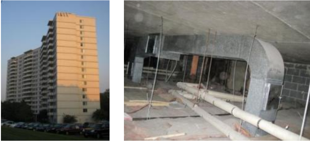
Figure 47. A 17-story multifamily building with large attic space
