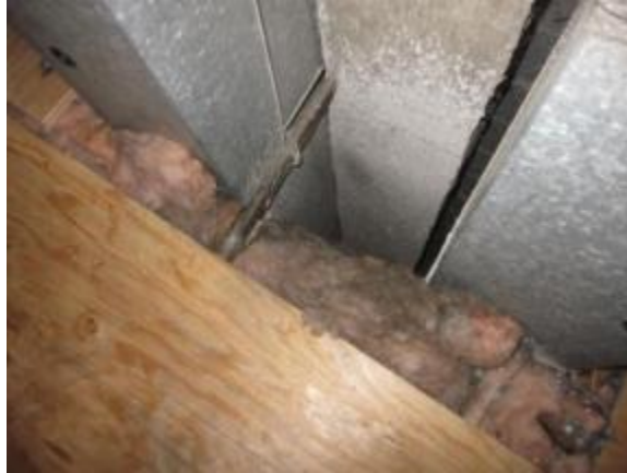
Figure 26. Mechanical chase in attic of a mid-rise apartment building
