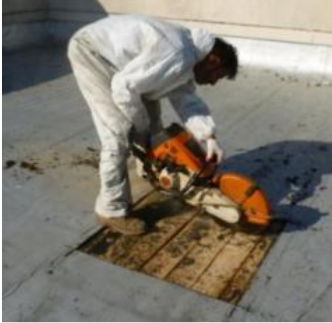
Access holes must be cut to access the attic
