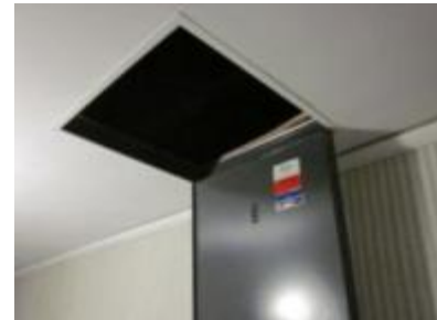
Figure 41. Attic access hatch
