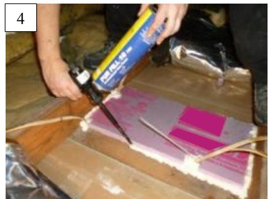
Figure 28. Step-by-step sequence for blocking an open soffit from attic side.
