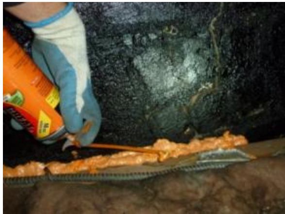
Expanding foam quickly seals the gap at the exterior wall
