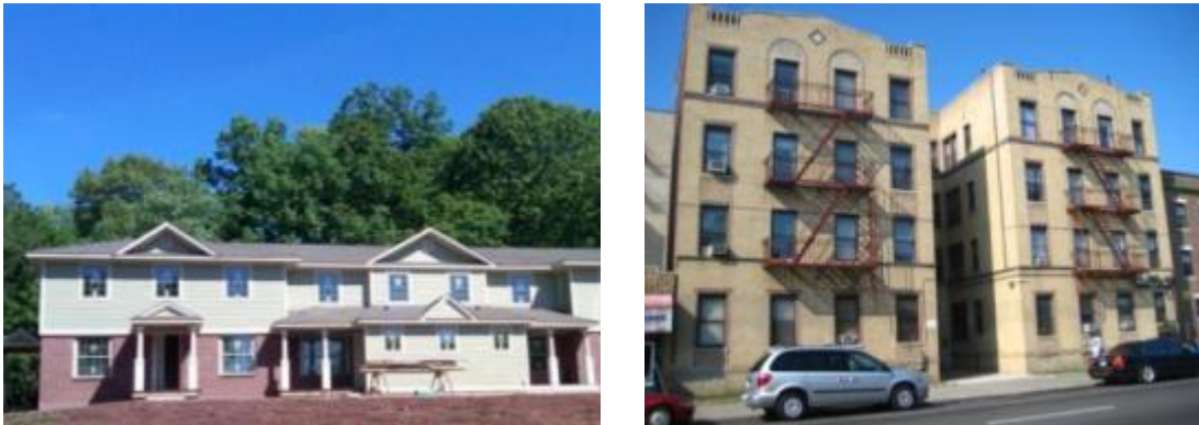
Figure 2. Examples of multifamily buildings
