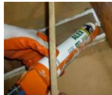
Figure 20. Caulk sealing small cracks
