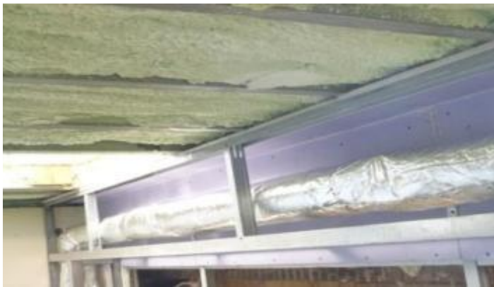
Figure 29. Soffit with continuous drywall at ceiling in a gut-rehab project
