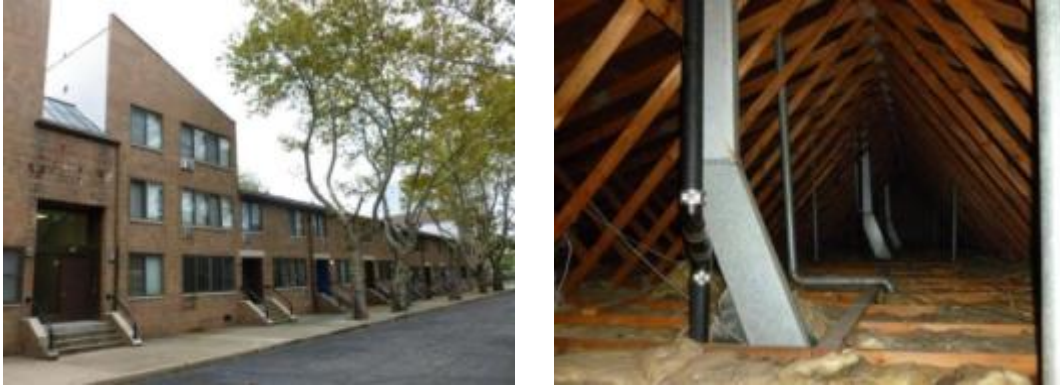
Figure 43. Shared attic for attached townhouses
