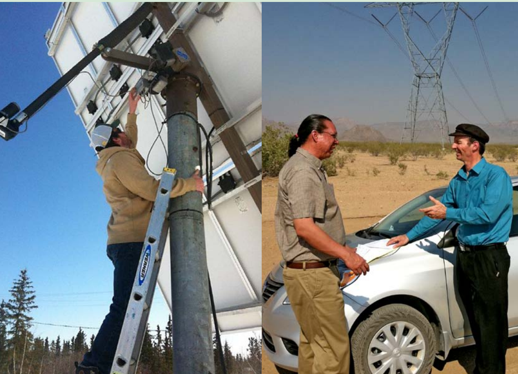
Left: During a START site visit, Alexander Dane of NREL repairs the tracking motor of the community-owned solar photovoltaic (PV) array in Venetie, Alaska. Photo by Brian Hirsch, NREL/PIX 20893. Right: Paul Dearhouse of Dearhouse Consulting and Kevin Davidson of the Hualapai Tribe Planning and Economic Development Department discuss utility-scale solar and wind project potential during a START site visit in Arizona. Photo by Bob Springer, NREL/PIX 21044.
