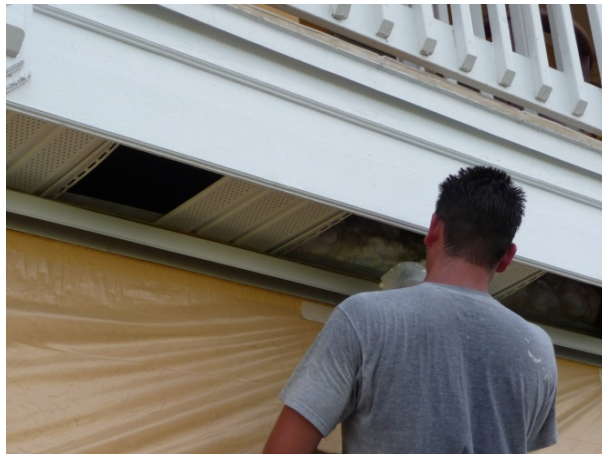
Figure 31. Opening to floor cavity is sealed by application of foam to create an insulating air barrier between each floor joist.
