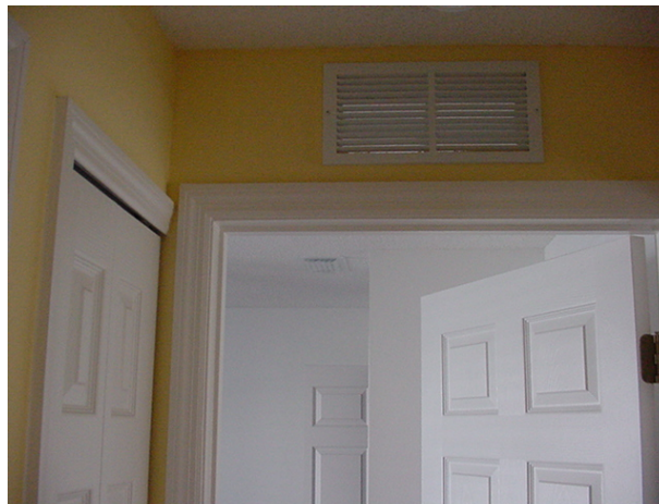
Figure 73. Through-the-wall return transfer from bedroom to hallway.
