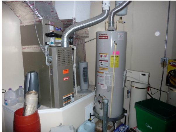
Figure 53. A gas furnace is located on a support platform used as the return plenum located inside a garage next to a gas water heater. Return leakage can depressurize the garage and interfere with proper venting of these atmospherically vented gas appliances.
