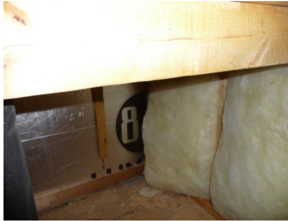
Figure 55. View inside a return plenum located in a second floor closet shows lack of effective duct air or thermal barrier. Attic air could be drawn down leaks in wall cavities and through the floor cavity, which is also well connected to an attic space.
