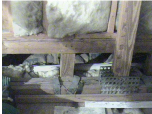
Figure 22. Close-up view of entry to open floor cavity.
