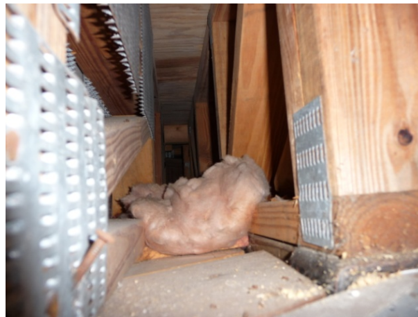
Figure 29. View from the vented eave cavity that is well-connected to second-story floor cavity.
