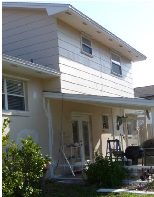
Figure 34. Second-story floor cavity has cantilevered section that was vented on the back side of home.
