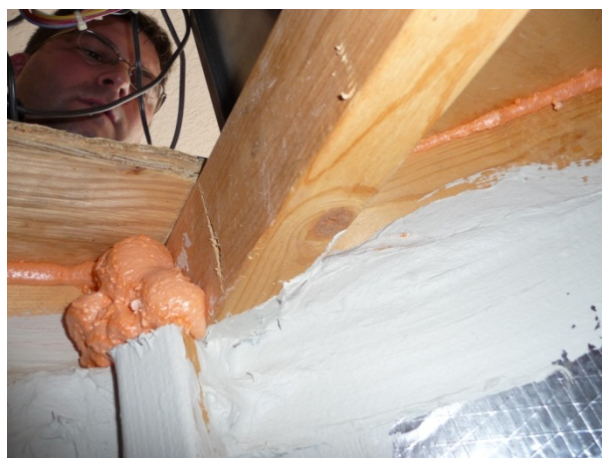
Figure 59. All seams in this support platform return plenum have been sealed using mastic.
