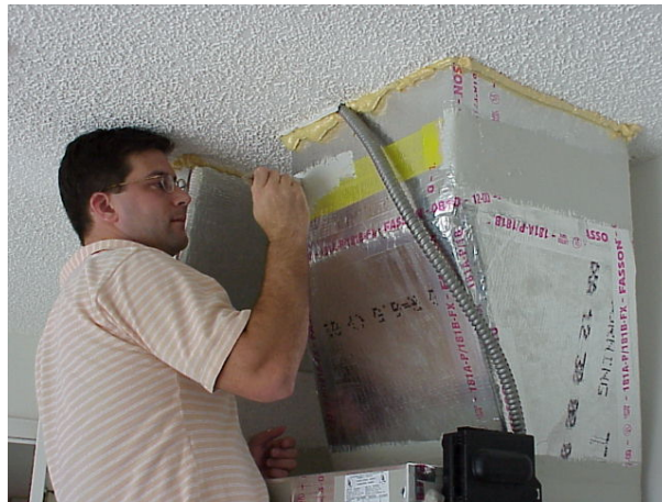
Figure 68. Supply plenum connection being sealed using foil tape, fiberglass mesh tape, and mastic.
