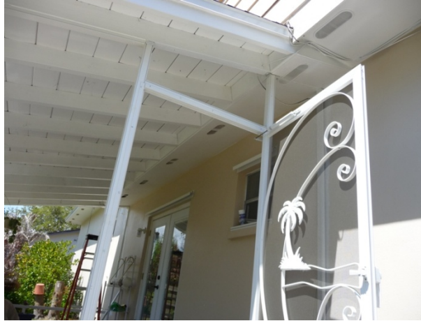
Figure 35. Oval shaped soffit vents can be seen on the underside of cantilevered floor section.
