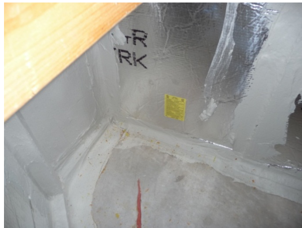
Figure 59. All seams in this support platform return plenum have been sealed using mastic.
