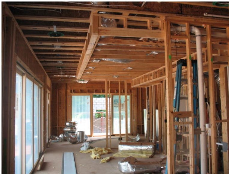
Figure 4. TaC Studios residence framing
