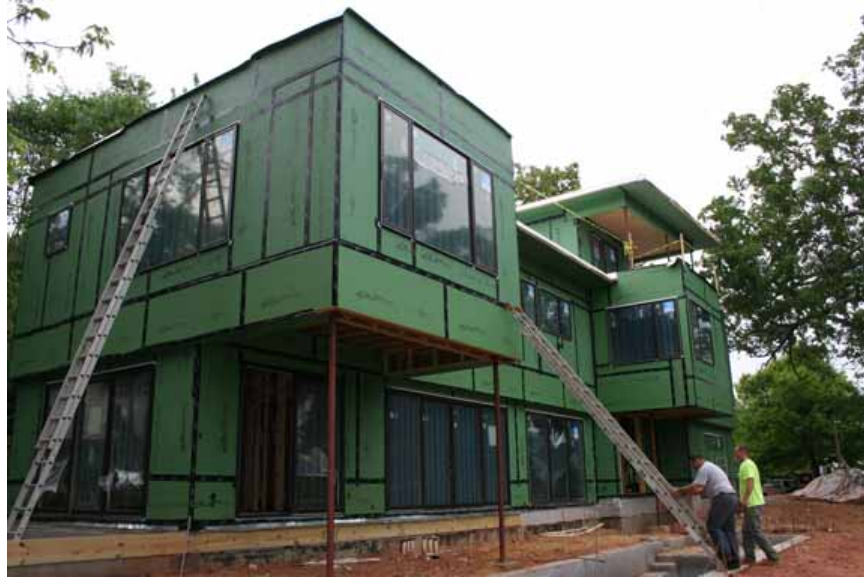
Figure 5. Taped exterior sheathing panels
