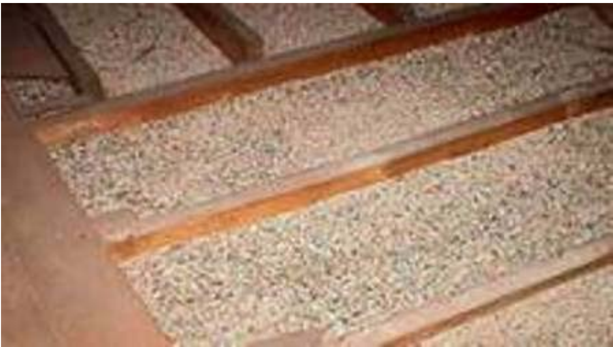
Figure 2. Vermiculite insulation between joists
