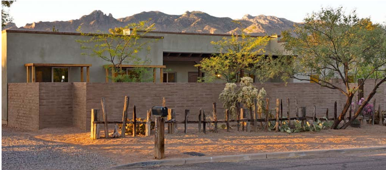
Figure 2. Completed S.E.E.D house
