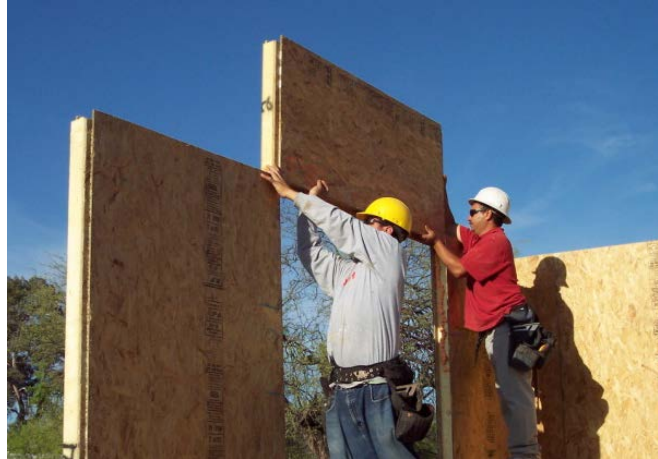
Figure 3. SIP wall installation
