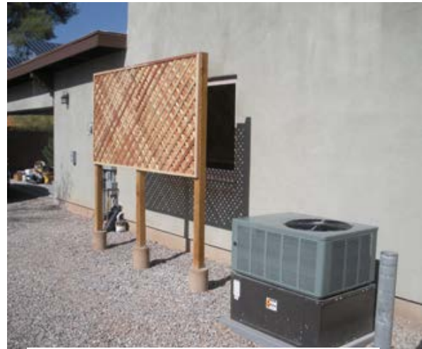
Figure 5. West elevation showing sun screen over window and air-to-water heat pump.
