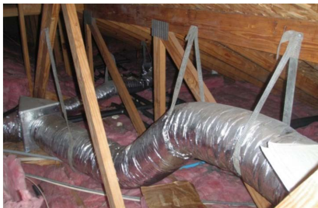
Figure 1. Traditional ductwork hung from attic rafters
