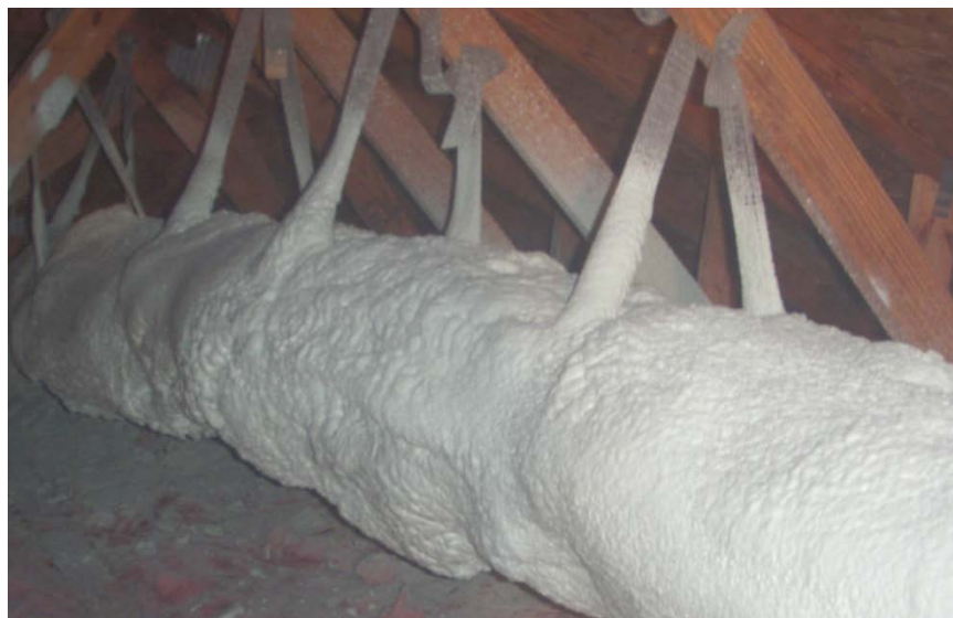
Figure 13. Finished encapsulated duct hung from roof deck
