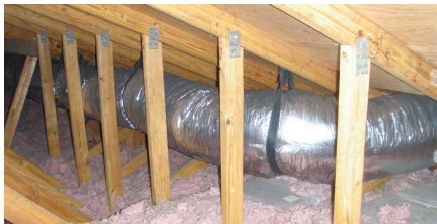
Figure 9. Return ductwork for House 2
