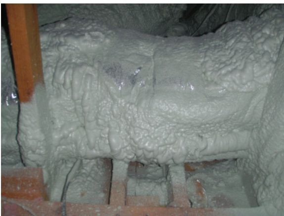
Figure 22. Varying thickness of ccSPF and interference from cross bracing
