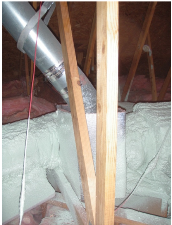
Figure 15. Baffling used to prevent ccSPF application on flue duct
