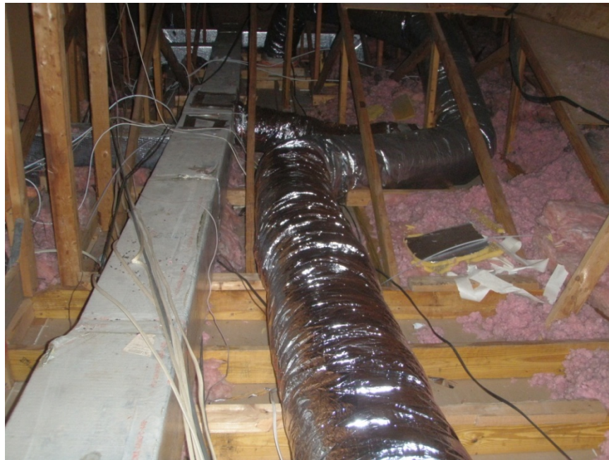
Figure 11. Duct reconfiguration at House 2
