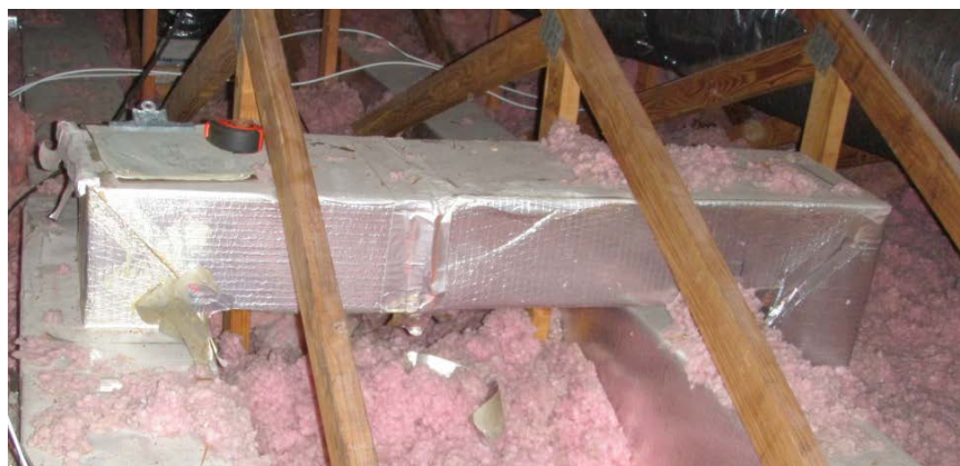
Figure 10. Supply ductwork jump over abandoned return ductwork
