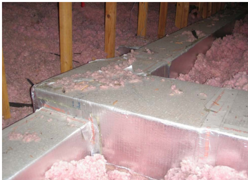
Figure 8. Supply ductwork for House 2
