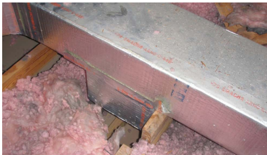
Figure 12. Open duct take-off at House 2
