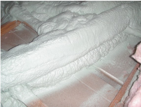
Figure 20. Ductwork well-sealed to sheetrock with ccSPF
