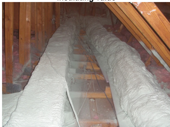
Figure 23. Varying application thicknesses shown on rectangular (left) and round (right) ducts
