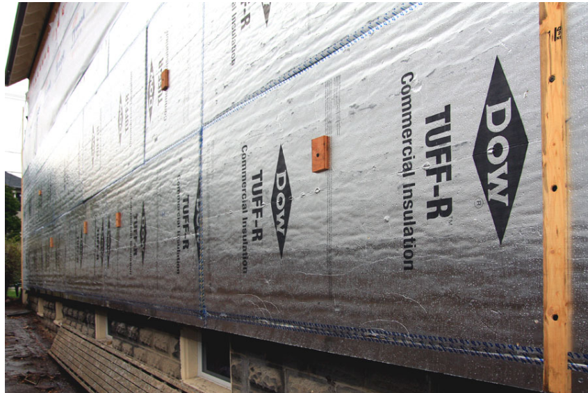
Figure 2. Insulating sheathing on the Belmont Two-Family
