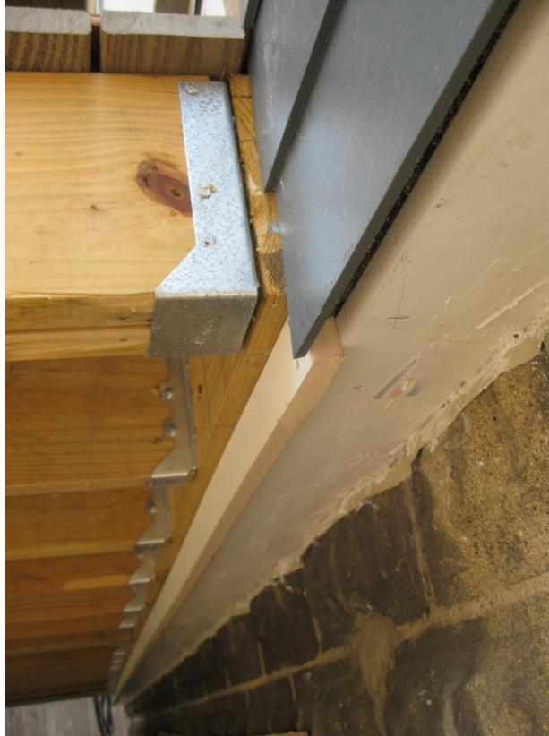
Figure 8. Belmont Two-Family porch deck attachment (from below)
