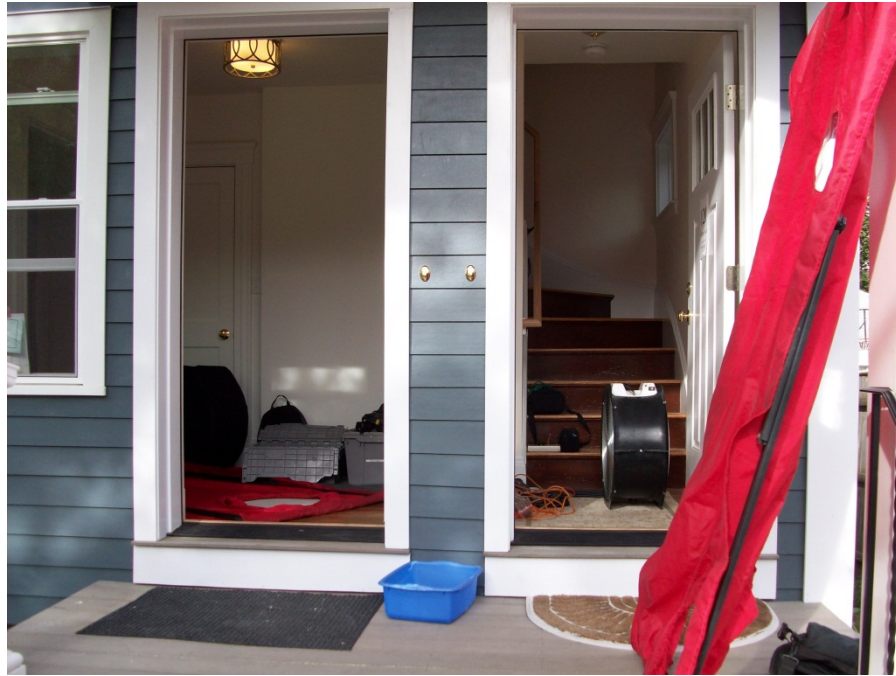
Figure 14. Belmont Two-Family: Setting up blower door testing
