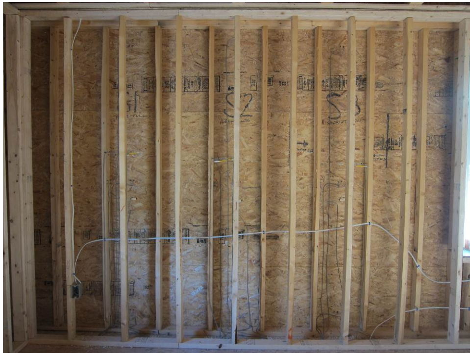
Figure 50. South test walls after installation of sensors, showing double-stud layout
