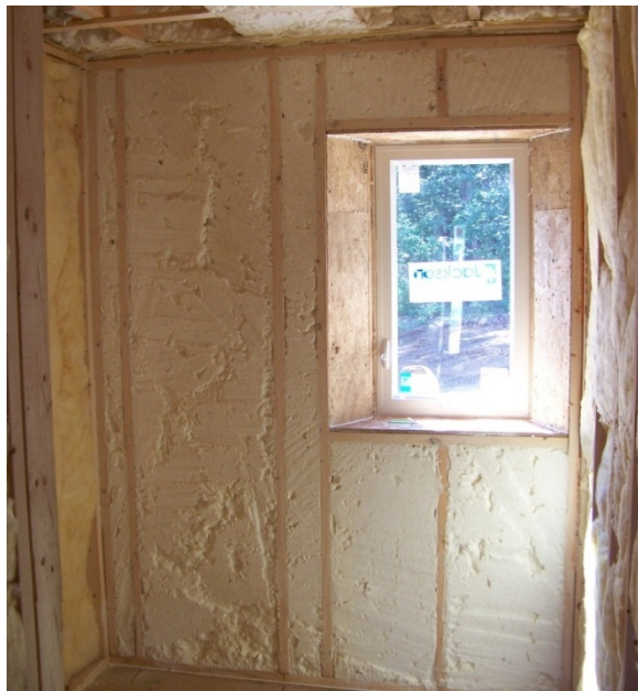
Figure 44. Typical installation of ½ lb/ft 3 spray foam in double-stud walls
