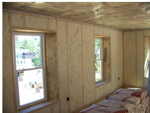
Figure 44. Typical installation of ½ lb/ft 3 spray foam in double-stud walls
