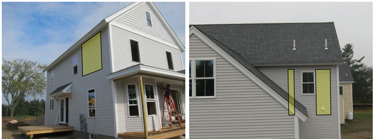
Figure 47. Test wall locations shown on exterior of house; south (L) and north (R) orientations
