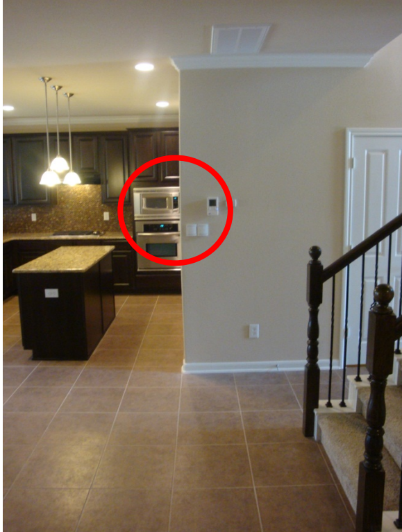
Figure 22. Location #1; first-floor temperature and RH measurement at the thermostat location
