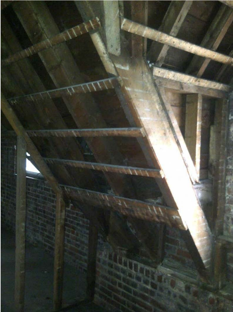
Figure 15: Original building – interior view of sloped roof
