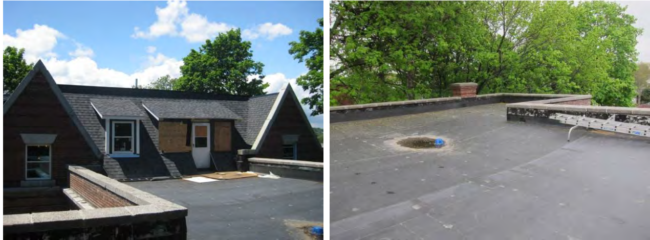
Figure 31. (L) Lower roof, showing upper roof; (R) upper roof
