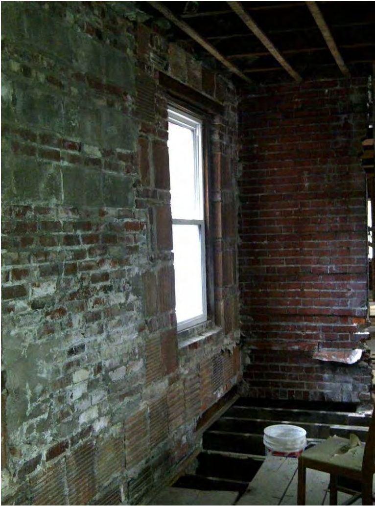
Figure 24: Addition - a typical window
