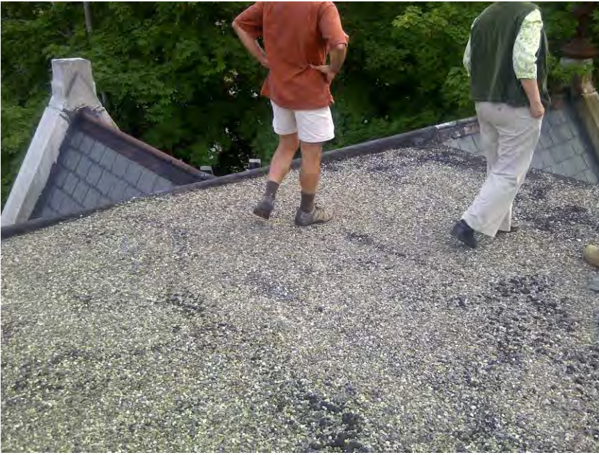
Figure 10: Original building – flat roof area
