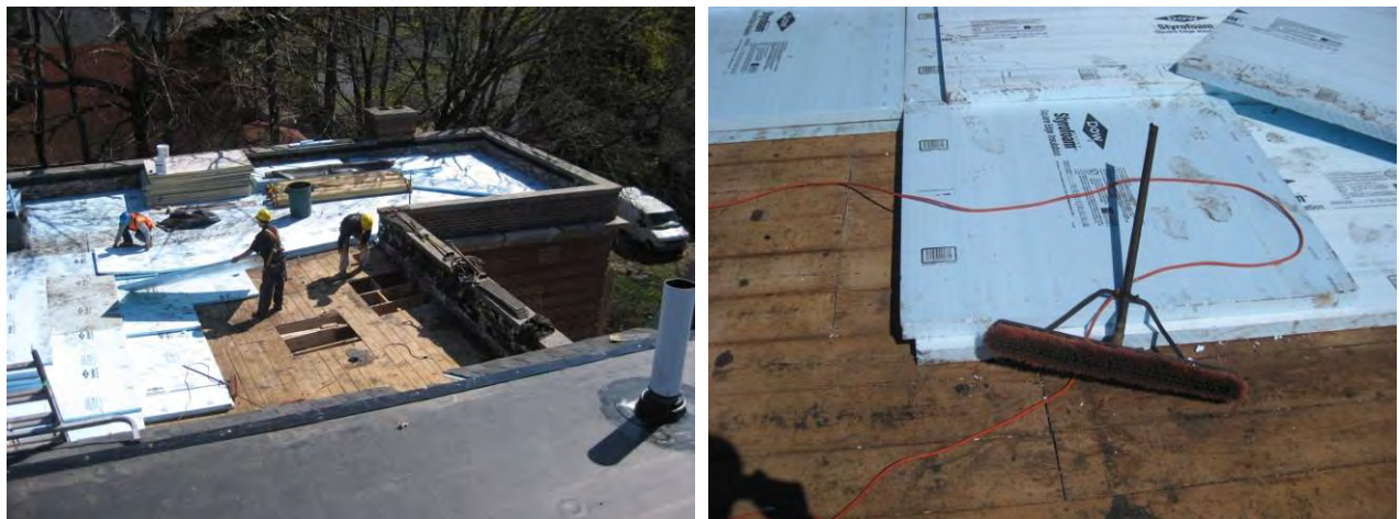
Figure 30. Insulation of lower roof, showing lack of air barrier at board sheathing
