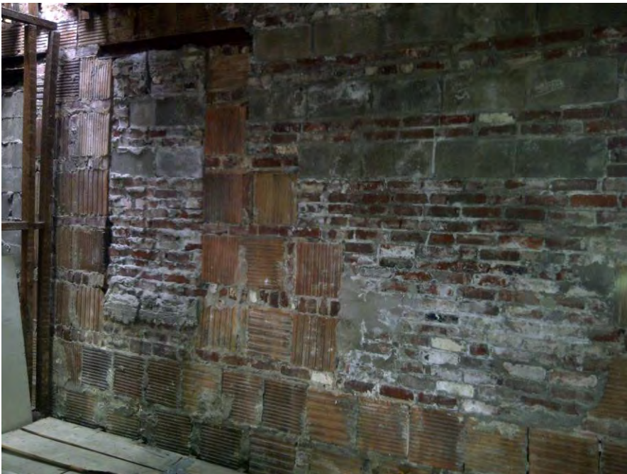
Figure 25: Addition – views of various interior materials used in masonry mass walls
