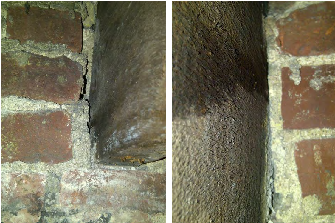
Figure 14: Original building - floor joist to masonry wall interface
