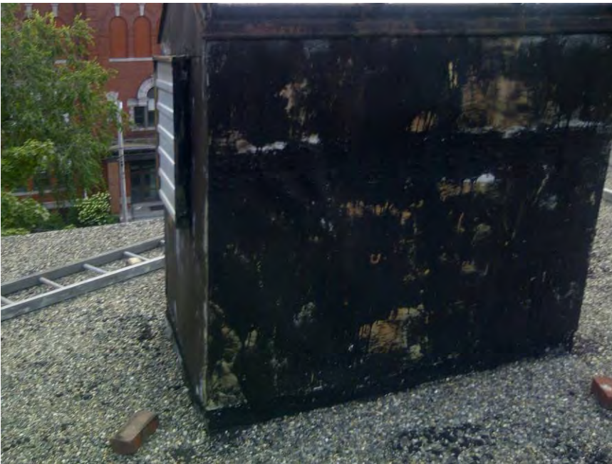
Figure 11: Original building – clerestory
