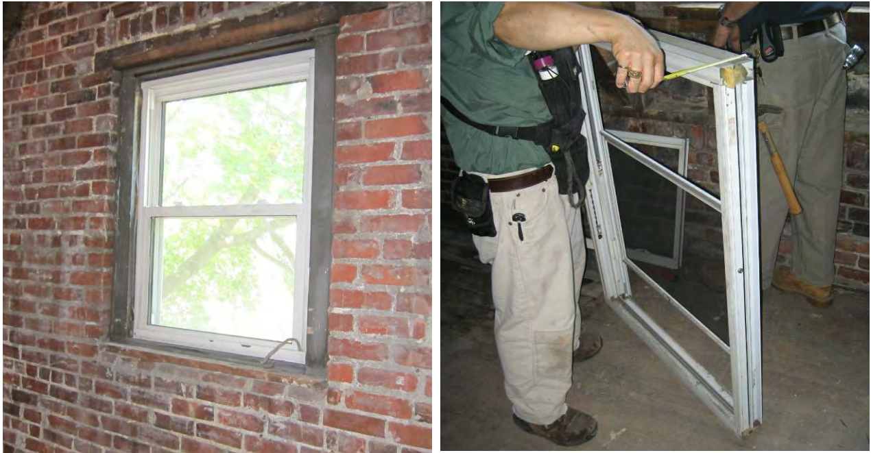
Figure 20. Existing vinyl double-glazed (clear) insert replacement windows
