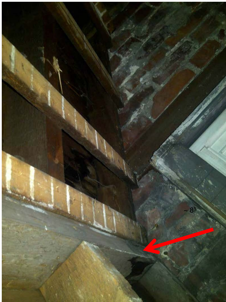
Figure 16: Original building – interior view of sloped roof
