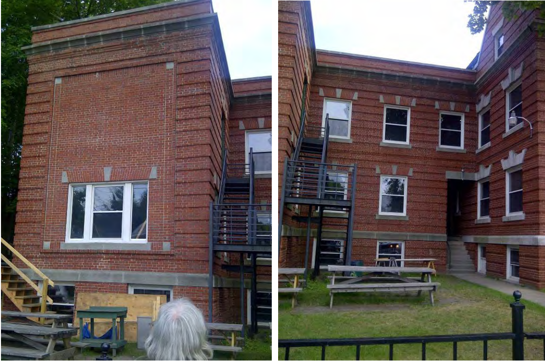
Figure 18: Addition - North Façade
