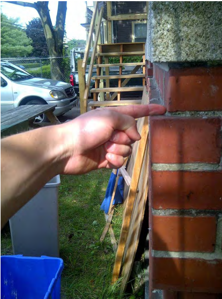
Figure 5: Original building – close up of brick courses
