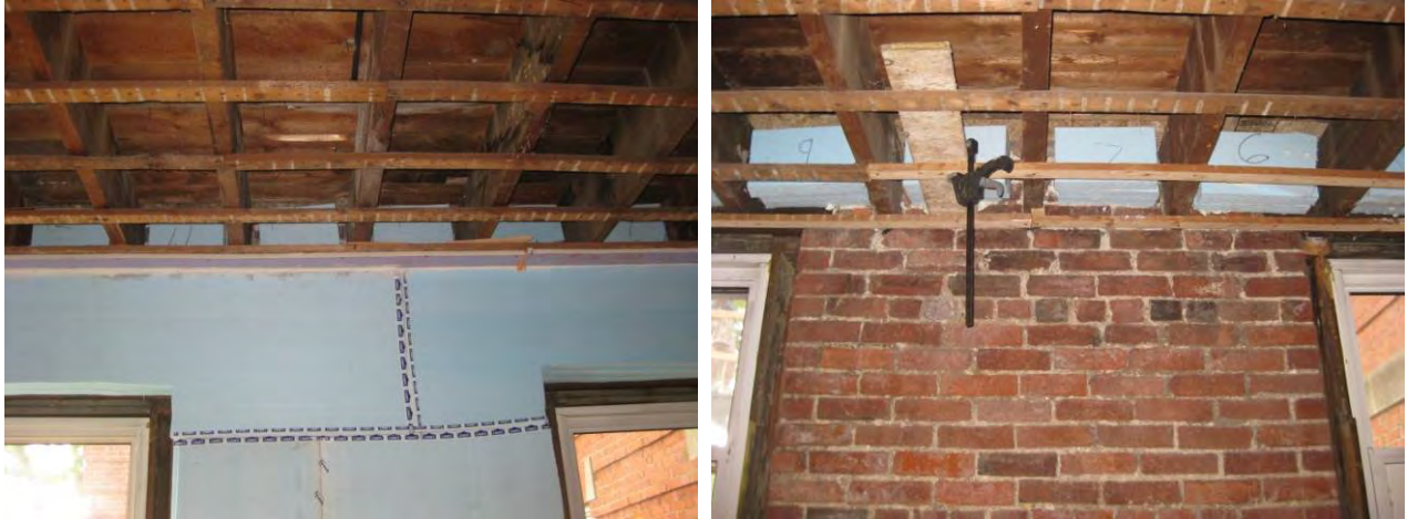
Figure 44. (L) Rim joist foam blocks; (R) close-up showing clamping jig
