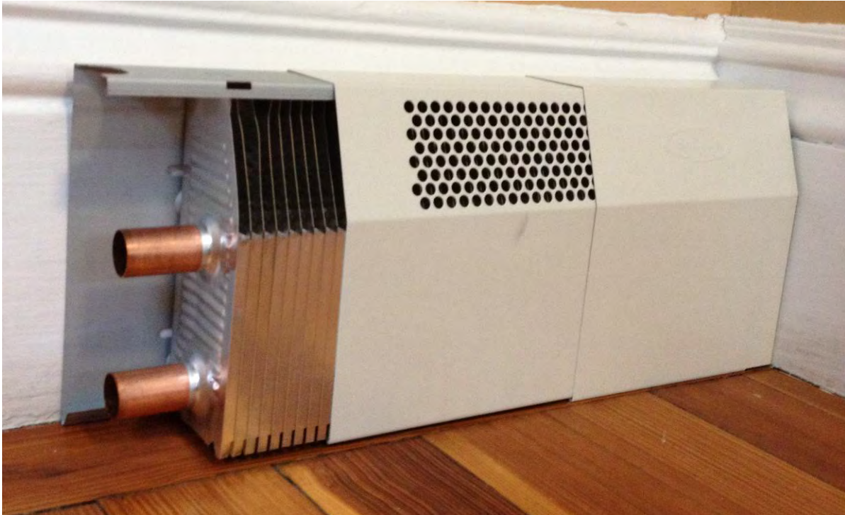
Figure 53. Smith Environmental HE2 high-capacity hybrid element
