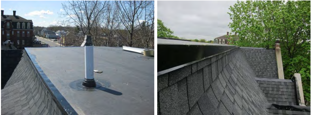
Figure 33. (L) Upper roof typical conditions; (R) upper roof edge detail
