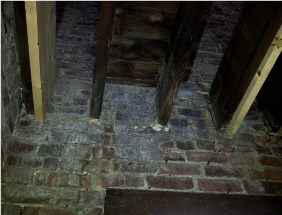
Figure 13: Floor joists set in masonry wall
