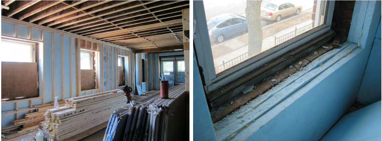
Figure 26. (L) Framing installed inboard of insulation; (R) conditions at window opening
