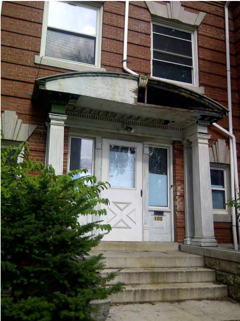
Figure 3: Original building –front entrance
