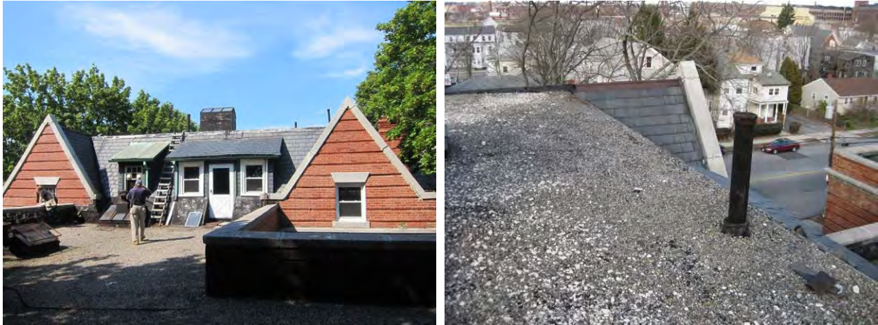
Figure 28. (L) Lower roof, showing upper roof; (R) upper roof
