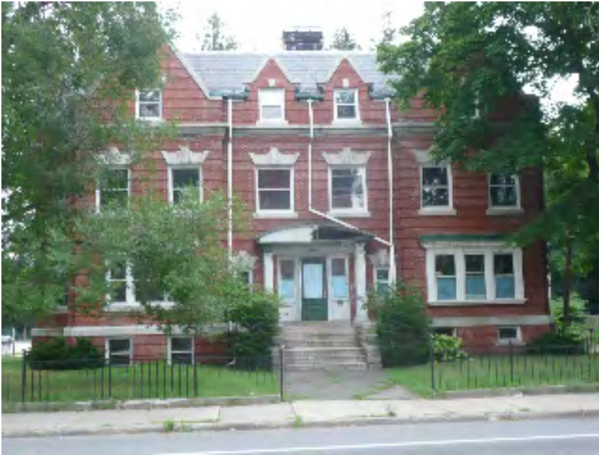
Figure 4: Original building – general view of building frontage.
