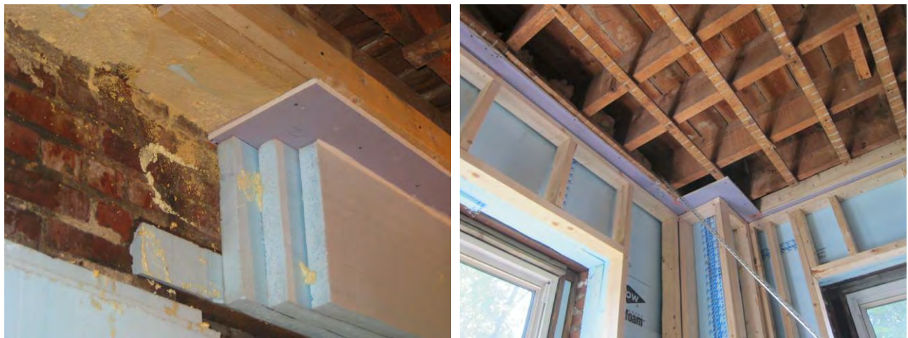
Figure 43. (L) Floor/ceiling fire separation gypsum board; (R) conditions after interior framing
