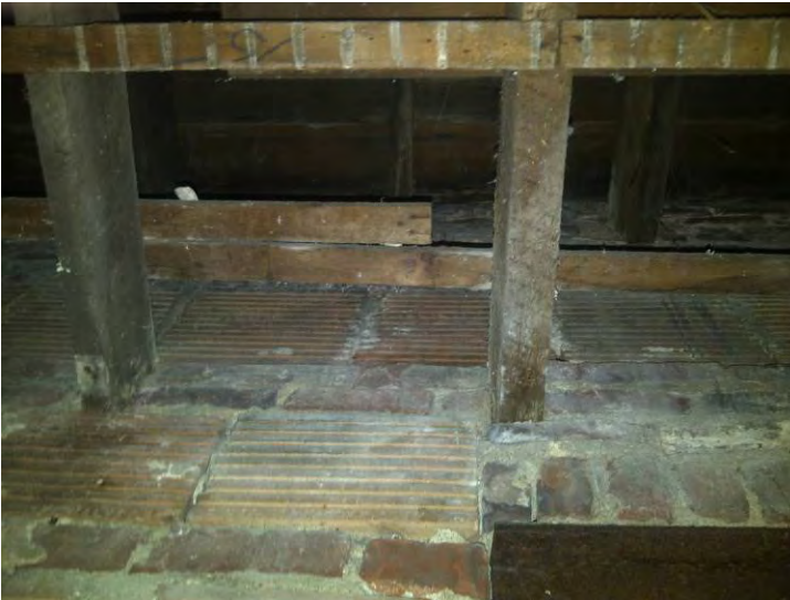
Figure 26: Addition – underside of roof
