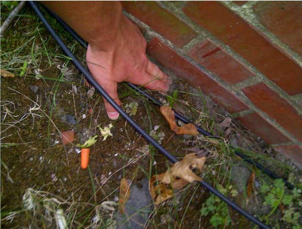
Figure 6: Original building – façade to ground interface
