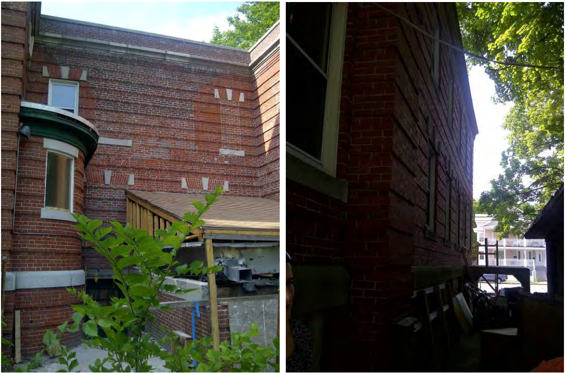
Figure 19: Addition - South Façade (left) and East Façade (right)
