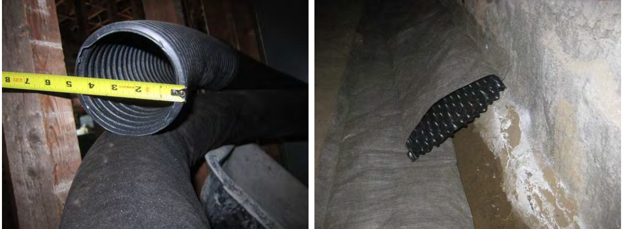
Figure 37. (L) 4 in. nominal corrugated drainage pipe; (R) low-profile radon vent mat
