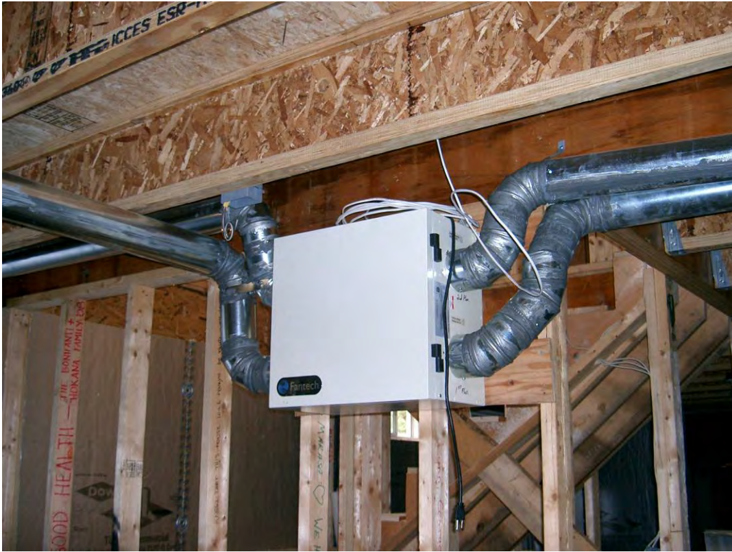
Figure 59. Proposed HRV installation example
