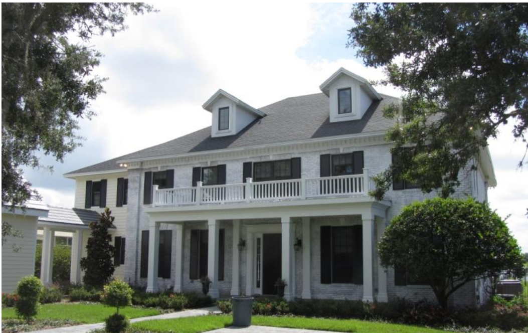
Figure 1. Front elevation (west) of the CEH post-retrofit
