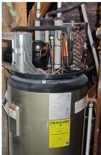
Figure 4. Cover removed from top of the monitored HPWH
