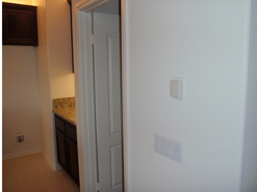
Figure 3. Indoor temperature and RH sensor in the kitchen and family room area
