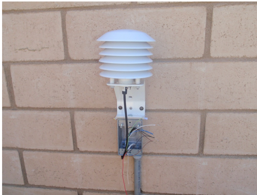
Figure 2. Outdoor temperature and RH sensor mounted on a privacy wall in the side yard
