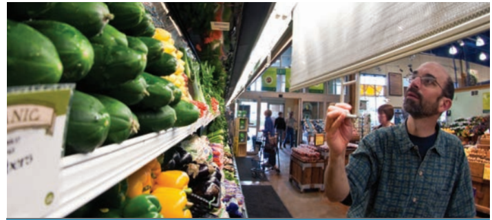
Whole Foods Market selected efficient lighting and night curtains for open produce cases. Photo by Pat Corkery, NREL 18596
