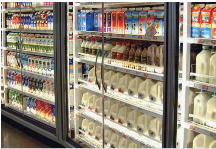
Whole Foods Market found that efficient refrigeration cases with doors do not present an inconvenience to shoppers. Photo by Jennifer Scheib NREL 18606
