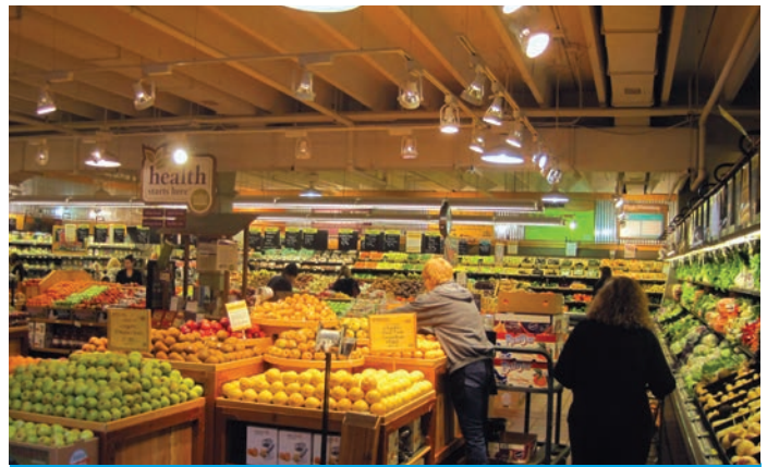
NREL and Whole Foods Market worked together to reduce produce area lighting power density at the Edgewater store to 0.8 W/ft 2 , a 20% decrease. Photo by Ian Doebber, 18609
