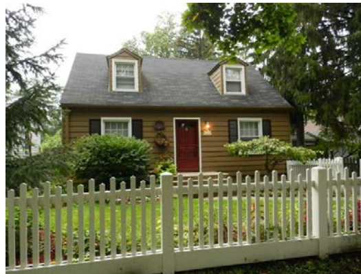
Figure 39. Cape Code style house
