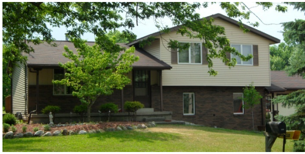
Figure 61. Split-level ranch style house 2
