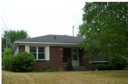
Figure 13. Ranch built after the 1960s
