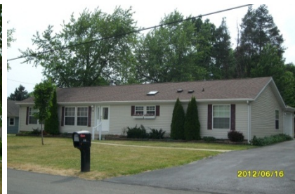
Figure 14. Ranch built after the 1960s
