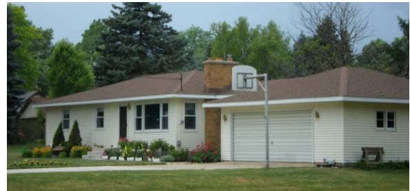
Figure 5. Example of a Ranch style house
