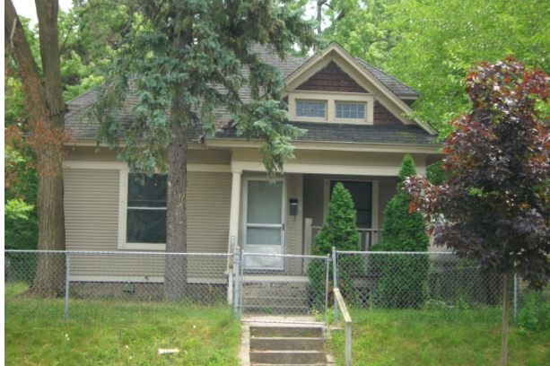
Figure 51. Bungalow style house
