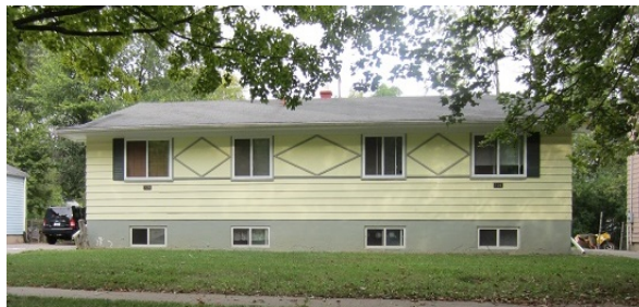
Figure 59. Raised Ranch style house
