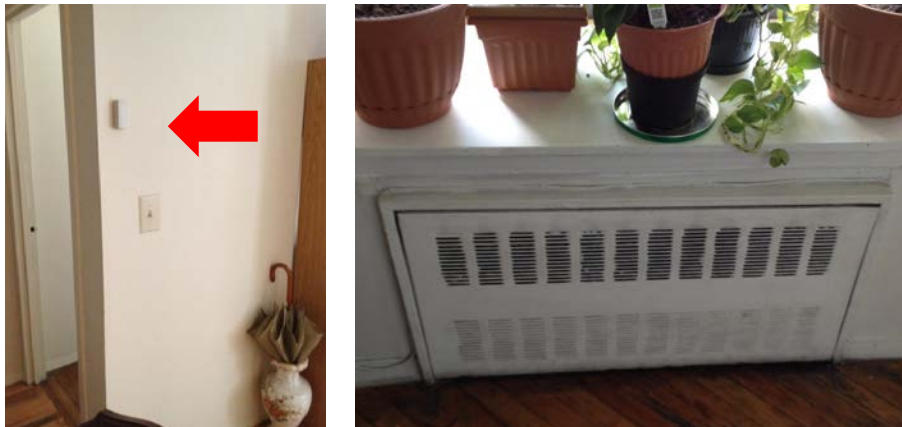
Figure 2. Typical wireless temperature sensor (left) and radiator (right)
